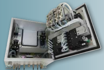
Tunneling machine control
