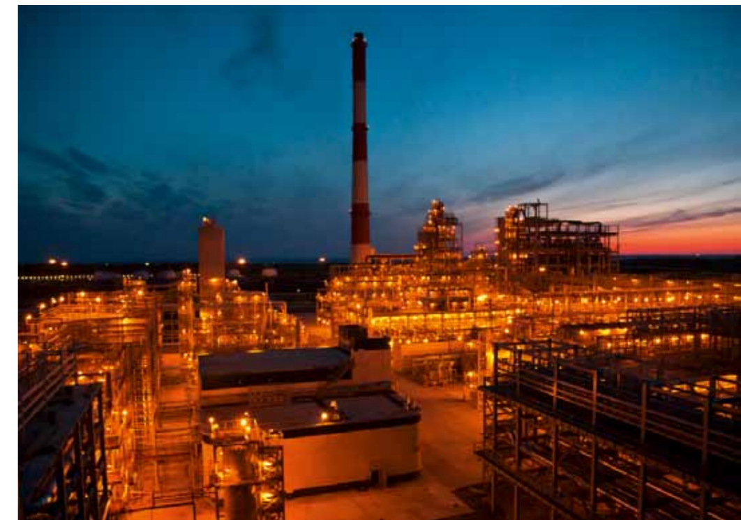
One of the world's largest refineries is located at Nizhnekamsk, Russia. The complex is scheduled to process 7 million metric tons of sour crude oil annually into a wide range of petrochemical products.
