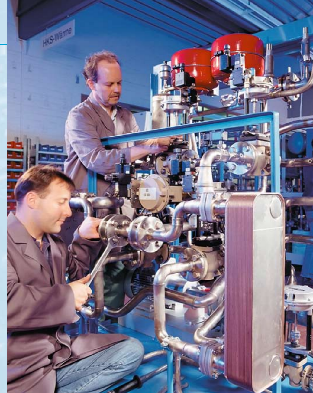
Final assembly of a heating and cooling system at Lauda.
