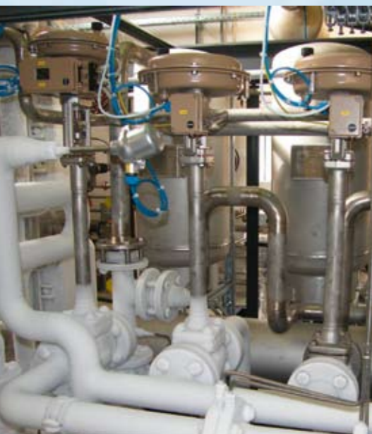
Long insulating sections protect the actuators against extreme temperatures in a cooling system.
