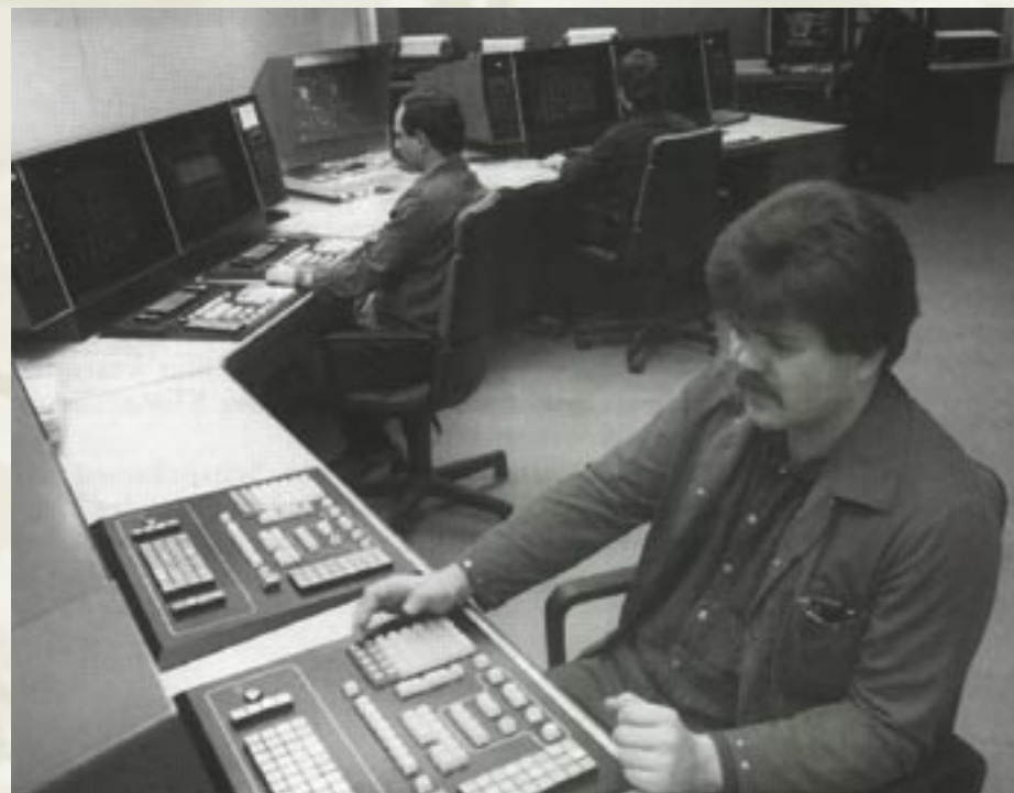
The workplaces in a control station with process control system around 1975. Control desks with monitors and keyboards had replaced the long walls of instruments.
