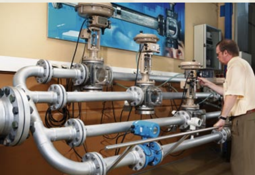
The positioners with bus communication are tested together with control stations and sensors under conditions similar to those in the process.
